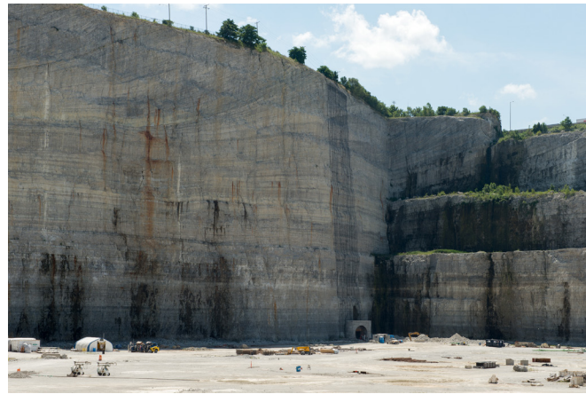
The Thornton Quarry has been mined all the way back to the 1860s, but it was an intriguing agreement made in 1998 that allowed Hanson Material Service the ability to mine it in preparation for the MWRD's Tunnel and Reservoir Plan.
