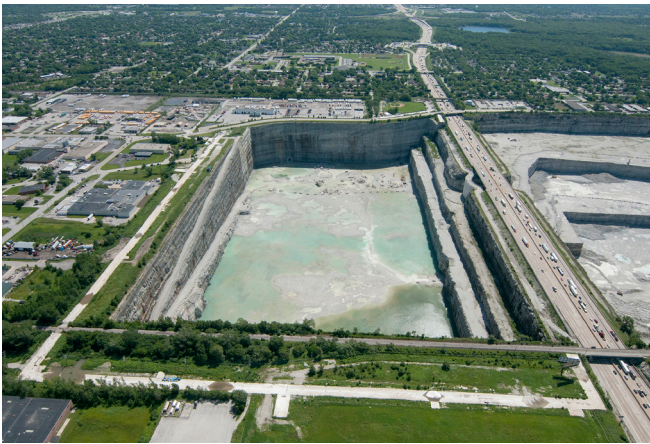
The world's largest reservoir, the MWRD's Thornton Composite Reservoir, shown looking east, can hold up to 7.9 billion gallons of water emanating from the tunnels on the east wall.
