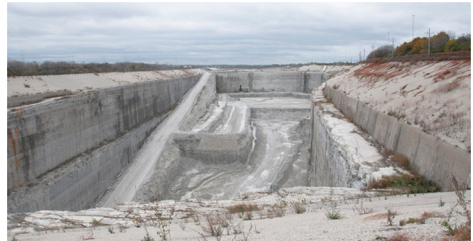
The McCook Reservoir, situated along the Stevenson Expressway (I-55) between the Des Plaines River and Chicago Sanitary and Ship Canal, will reduce pollution in the Chicago Area Waterways System by holding excess water before it can be treated. It will also provide flood relief for a service area more of more than 250 square miles.
