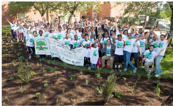
Students, staff and volunteers stand in a newly built rain garden on the playground at Pershing East Elementary School. The construction was part of the Water Environment Federation's (WEF's) 88th Annual Technical Exhibition and Conference. A 1,000 sq. ft. section of the property was replaced with native plantings to help relieve stormwater runoff. Each year, dozens of WEFTEC® participants arrive to their destinations early to participate in a service project.
