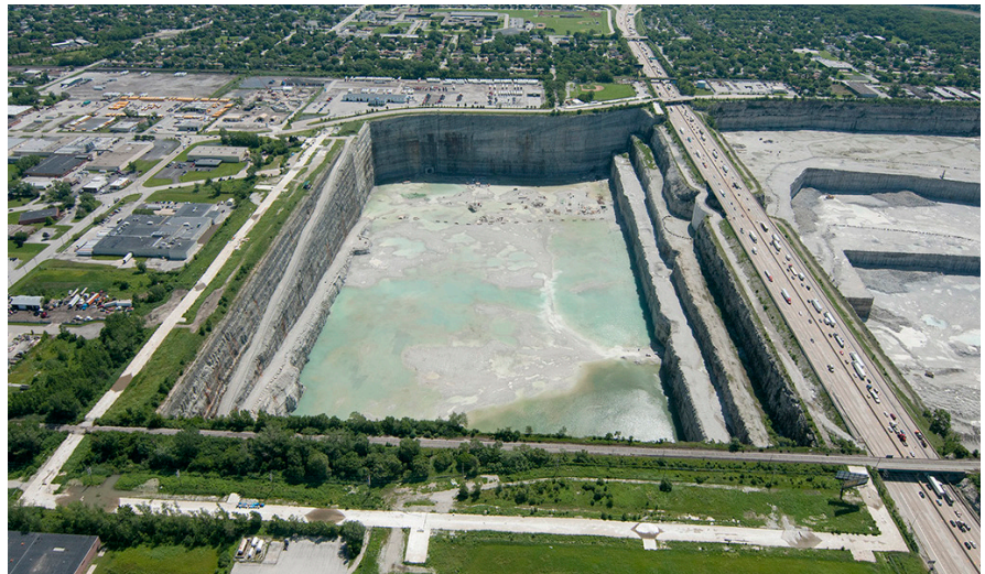
The world's largest reservoir, the Thornton Composite Reservoir, shown looking east, will hold 7.9 billion gallons of water emanating from the tunnels on the east wall.
