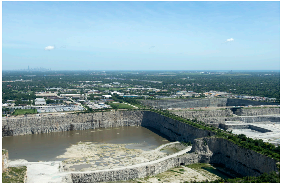
The Thornton Transitional Reservoir along I-294 in the south suburbs will operate adjacent to the Thornton Composite Reservoir to provide a total of 12.4 billion gallons of storage capacity for combined sewage and stormwater.
