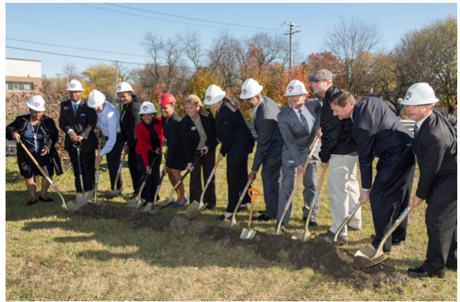
Public officials dig up ceremonial soil to signify the beginning of construction on 33 acre-feet of storage and a new 36" relief sewer in Westchester. The Mayfair Reservoir Expansion project will be completed next year.
