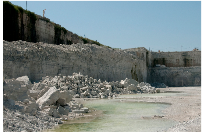
Stage 1 of the McCook Reservoir located on Interstate 55 is scheduled for completion in 2017 and will be able to contain 3.5 billion gallons of combined sewage. When fully functional in 2029, it will be able to capture and store 10 billion gallons. It will provide $90 million per year in flood control benefits to 3.1 million people living in 37 communities.
