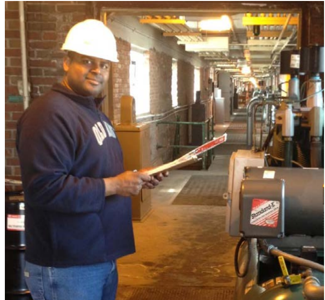
MWRD associate mechanical engineer WaShawn Brooks reviews upgrades made on an air compressor system at the Calumet Water Reclamation Plant in Chicago.
