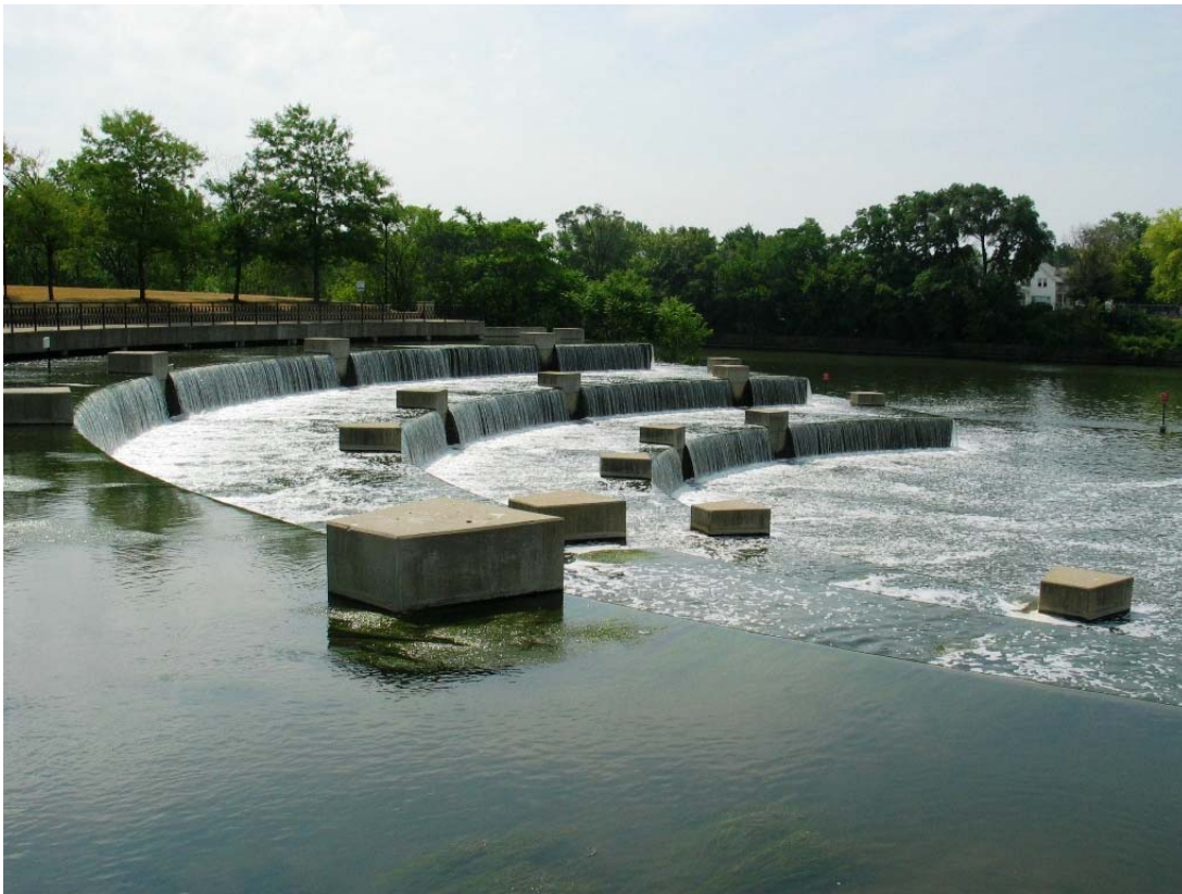
Figure 6. SEPA (Sidestream Elevated Pool Aeration) Station.
