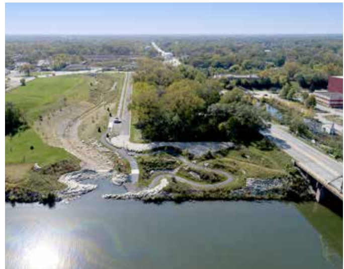
The Robbins Heritage Park and Midlothian Creek Restoration Project provides critical drainage for an area with no existing stormwater infrastructure. The project began with the creation of a diversion channel that connects flow to the Cal-Sag Channel with stone armoring along the channel waterline, a trail, waterfront access and a scenic backdrop.
