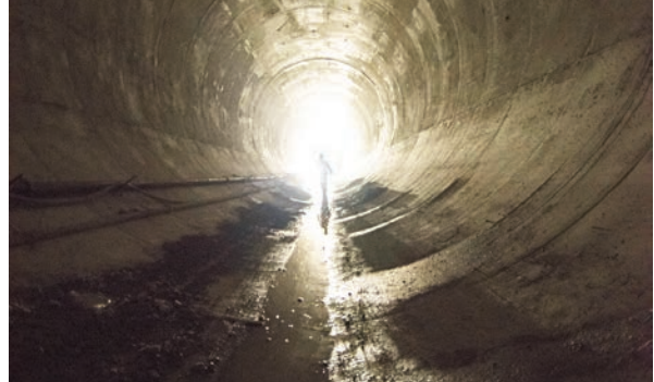
Tunnel and Reservoir Plan (TARP) captures sewage and stormwater during heavy rains to prevent sewer overflows, holding water until it can be treated.
