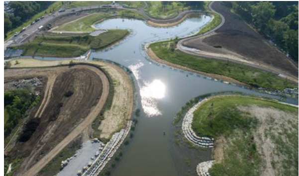
Flood control reservoirs , which temporarily store water from rivers and streams during storms.
