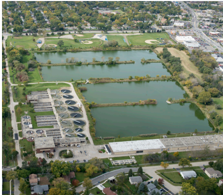
Hanover Park Water Reclamation Plant
