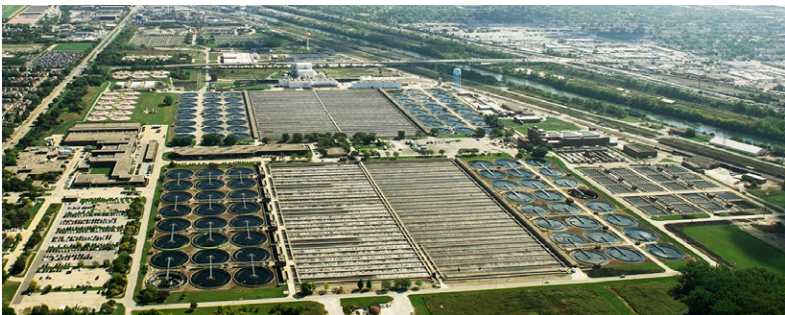
Stickney Water Reclamation Plant
