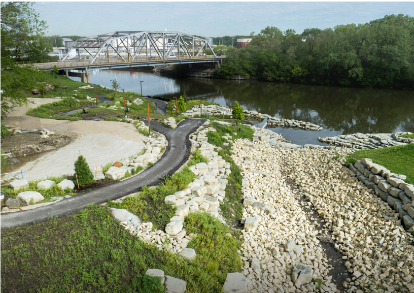
The diversion channel for the Midlothian Creek Flood Control Project in Robbins that the District helped fund is an example of a stormwater partnership project directly supporting municipalities in Cook County to address localized flooding and drainage concerns.
