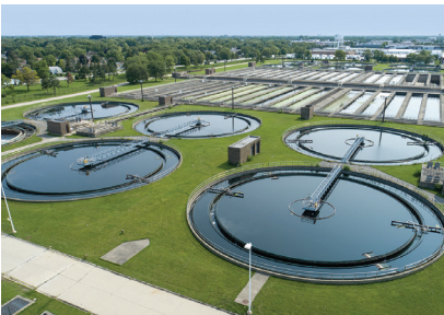
The James C. Kirie Water Reclamation Plant in Des Plaines treats an average of 52 million gallons of wastewater per day.
