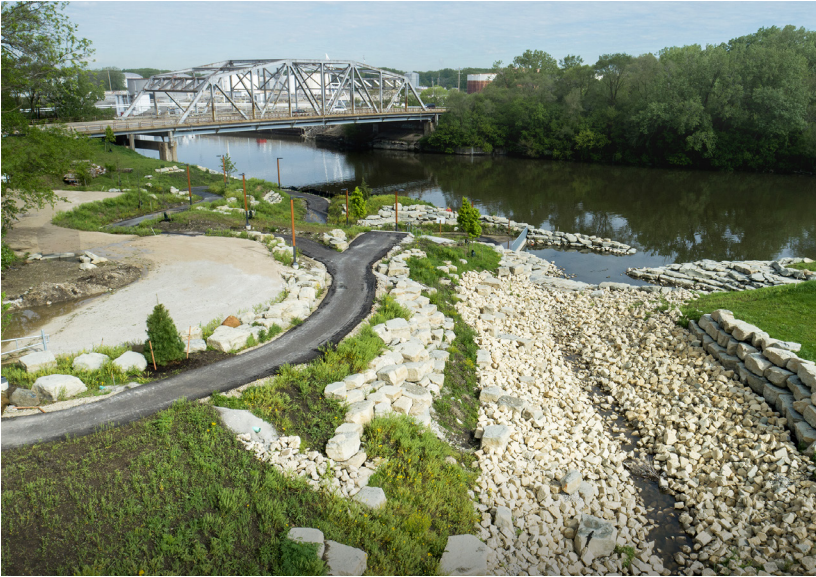
The diversion channel for the Midlothian Creek Flood Control Project in Robbins that the District helped fund is an example of a stormwater partnership project directly supporting municipalities in Cook County to address localized flooding and drainage concerns.
