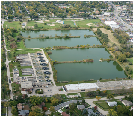
Hanover Park Water Reclamation Plant
