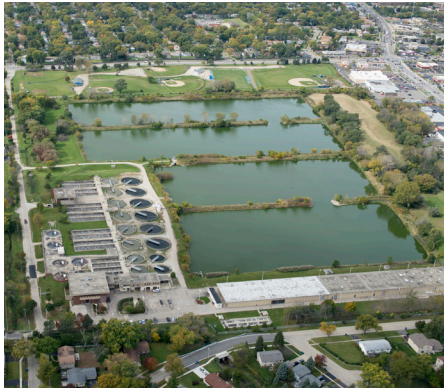
Hanover Park Water Reclamation Plant
