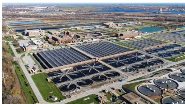
The Calumet Water Reclamation Plant is one of seven wastewater treatment facilities which serves residents and businesses in the southern portion of Cook County.
