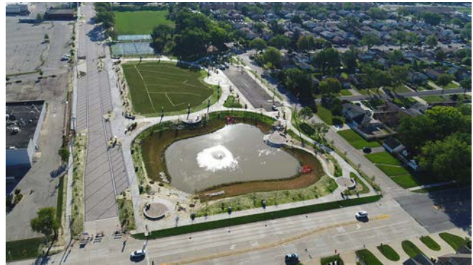
The Golf Mill Park stormwater project in the Village of Niles utilizes green infrastructure elements and permeable pavement to mitigate flooding and to improve local water quality.
