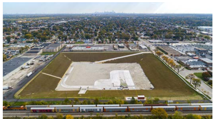
The District completed construction of the Addison Creek Reservoir and formally opened it at a ribbon cutting in August 2023.
