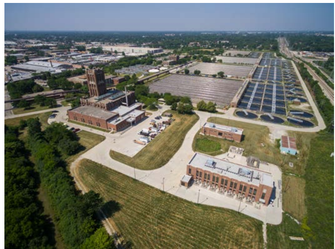
The O'Brien Water Reclamation Plant serves over 1.3 million people in communities north of downtown Chicago and features the largest ultraviolet disinfection facility for a wastewater plant in the United States, with a capacity to treat over 450 million gallons per day.
