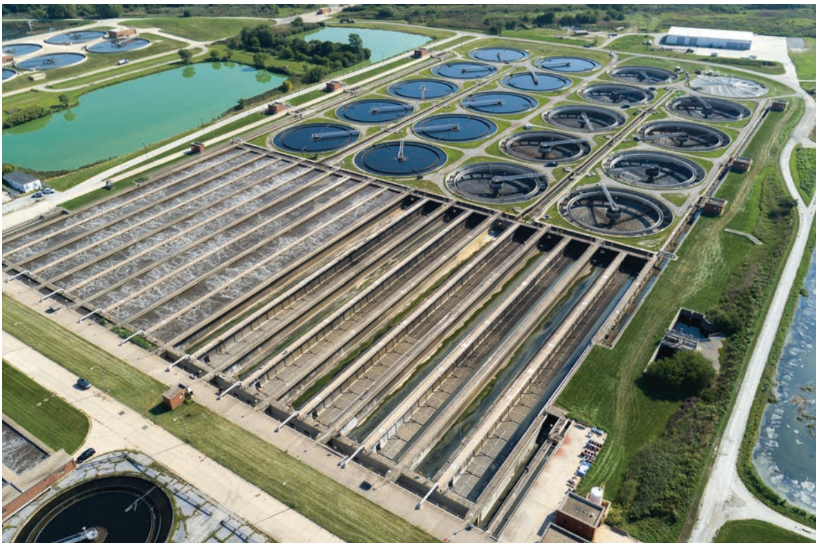
LEFT: Aerial views of Battery E1 at the Calumet Water Reclamation Plant (WRP) while the tanks were empty for maintenance in 2022.
