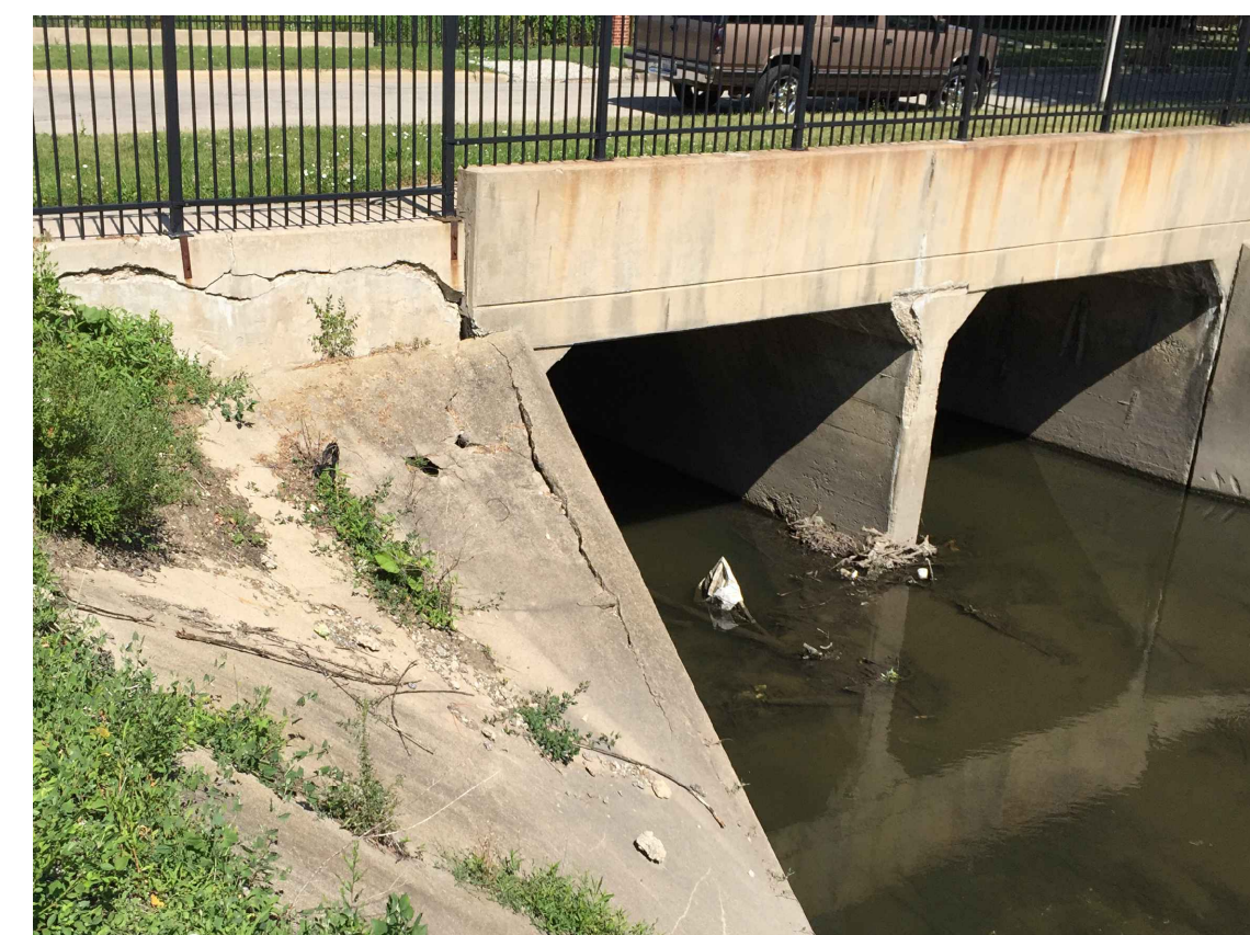
32ND AVENUE BRIDGE UPSTREAM FACE
