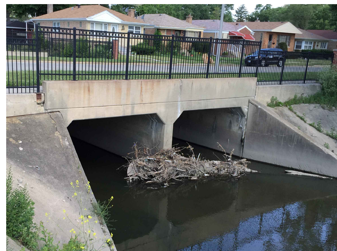
31ST AVENUE BRIDGE UPSTREAM FACE
