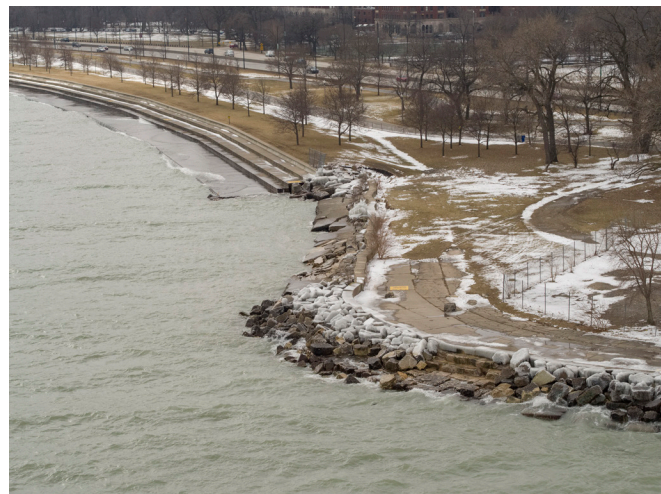
The MWRD will fund much needed lakefront restoration caused by high lake levels and damaging waves that occurred during major storms in January 2020.
