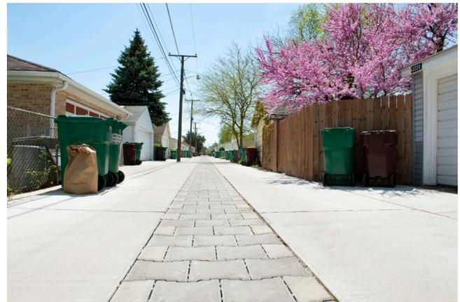
*A green alley in Berwyn, funded by the MWRD, collects precipitation where it falls by detaining and partially infiltrating runoff to prevent it from overwhelming sewers and flooding communities. The MWRD will contribute additional funds to expand green alleys in Berwyn, among other community projects in 2021.*
