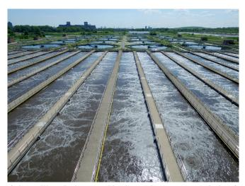
Calumet Water Reclamation Plant's secondary aeration tanks benefit from brewery waste high in readily biodegradable carbon that serves as food for phosphate accumulating organisms that remove excess nutrients from the water and lead to cleaner water downstream.
