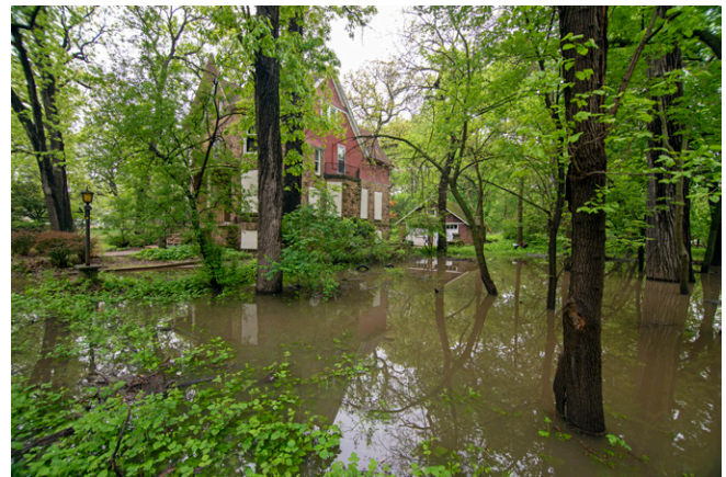
After repeated flooding incidents, homeowners and communities don't feel like they have a way out. A program offered by the MWRD can provide funding towards the purchase of these homes.
