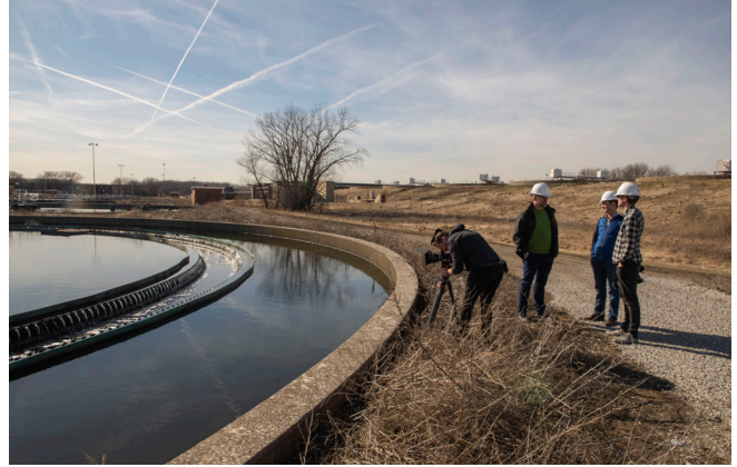
International filmmakers descended on the Stickney Water Reclamation Plant to film the MWRD's dynamic process to treat up to 1.44 billion gallons of water per day while working to recover resources from the treatment process.
