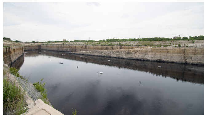
McCook Reservoir Stage I fills to hold up 3.5 billion gallons along with 1.6 billion gallons in the adjoining tunnels that feed into it. The water is held there until the MWRD can treat it. That untreated water formerly overwhelmed local sewers and overflowed into local waterways.
