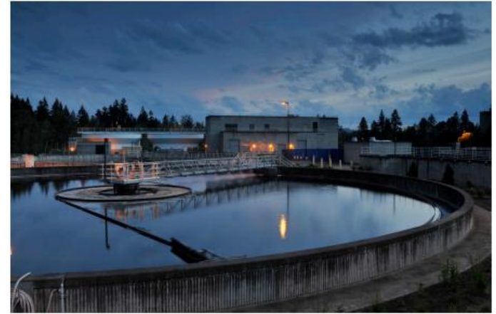
▲ Rock Creek AWWTF
