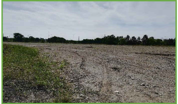
October, site cleared and ready for biosolids.
