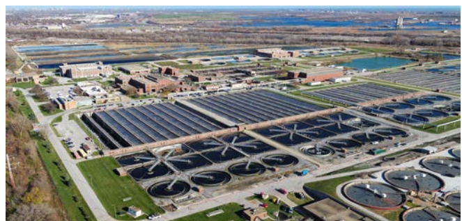
The Calumet Water Reclamation Plant is one of seven wastewater treatment facilities which serves residents and businesses in the southern portion of Cook County.
