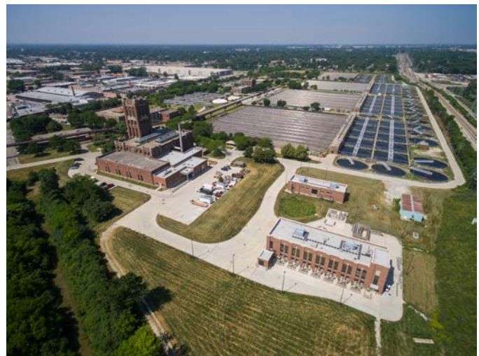
The O'Brien Water Reclamation Plant serves over 1.3 million people in communities north of downtown Chicago and features the largest ultraviolet disinfection facility for a wastewater plant in the United States, with a capacity to treat over 450 million gallons per day.
