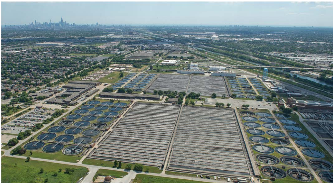
Stickney Water Reclamation Plant
