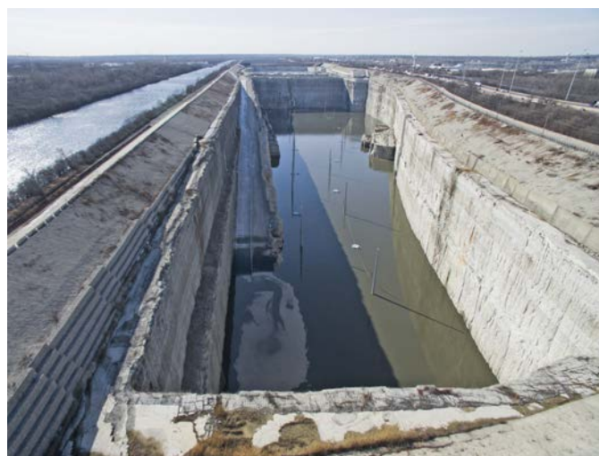
The McCook Reservoir is located along the Stevenson Expressway between the Des Plaines River and Chicago Sanitary and Ship Canal. It will serve 3.1 million people in 37 communities, including most of the City of Chicago.
