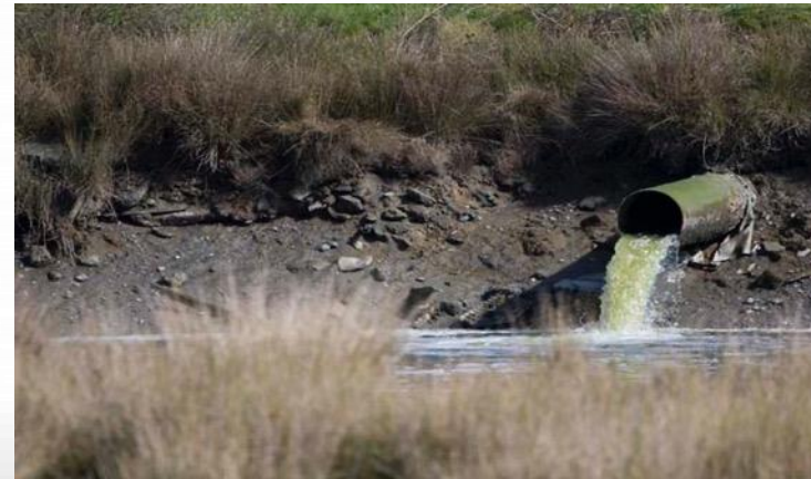
WWTP effluent outfall
