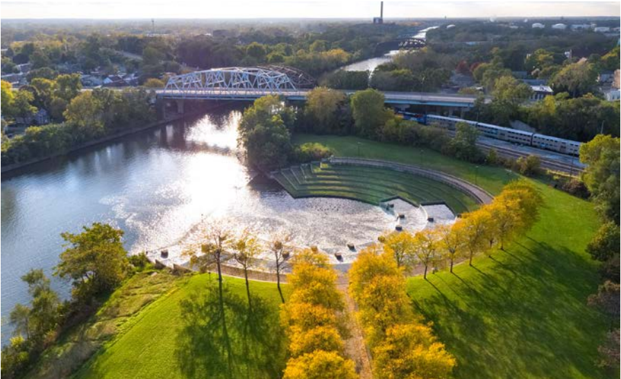
The MWRD's Sidestream Elevated Pool Aeration station 3 in Blue Island has a capacity of 300+ million gallons of water/day and utilizes 5' waterfalls to pump oxygen into the water to aerate the channel and create a thriving habitat for fish and wildlife.
