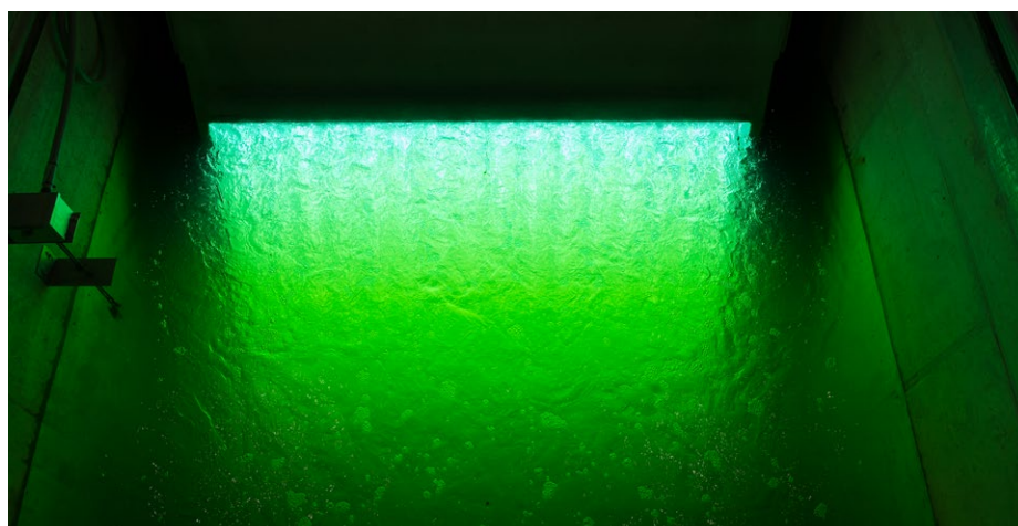
Powerful UV light neutralizes microbes in the water before it is released from the O'Brien WRP. Although UV the light itself is invisible, the 896 bulbs in the disinfection facility emit green light in the visible spectrum.
