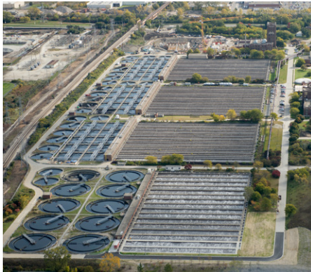
O'Brien Water Reclamation Plant
