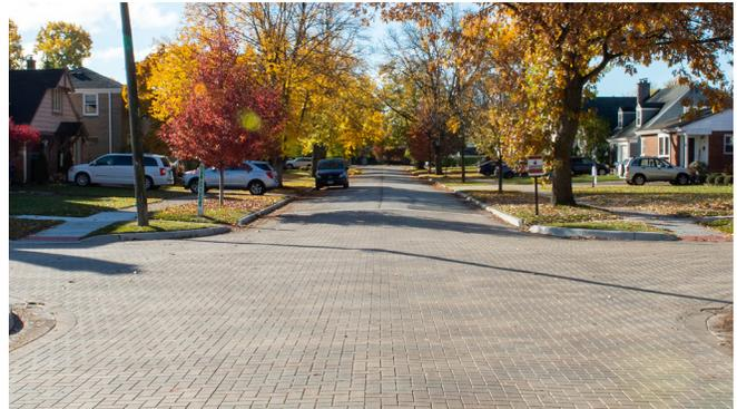
*Before and After: A new permeable intersection at Monroe Avenue and Sherwood Road is one of three green permeable intersections the Village of La Grange Park has converted thanks to MWRD support and funding.*
