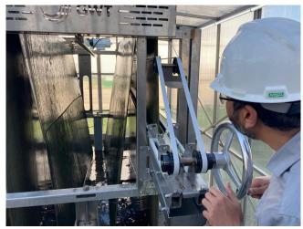
A revolving algal biofilm system naturally uptakes phosphorus and nitrogen from wastewater streams to support the growth of algae through photosynthesis and energy from the sun. The MWRD is using this process to remove nutrients from the waste stream without the use of inorganic chemicals or energy-consuming aeration, which is the traditional means of nutrient removal.
