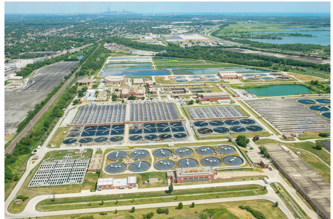
The Calumet Water Reclamation Plant, 400 E. 130th St., in Chicago, has continued its sterling reputation for transforming wastewater into clean water from its service area that covers 300 square miles.
