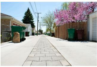
A green alley in Berwyn, funded by the MWRD, collects precipitation where it falls by detaining and partially infiltrating runoff to prevent it from overwhelming sewers and flooding communities. The MWRD will contribute additional funds to expand green alleys in Berwyn, among other community projects in 2021.
