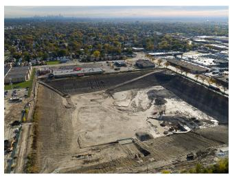
One of the many projects highlighted in the MWRD's 2022 budget is the MWRD's Addison Creek Reservoir, which along with Addison Creek Channel improvements, will protect west suburban communities from flooding.
