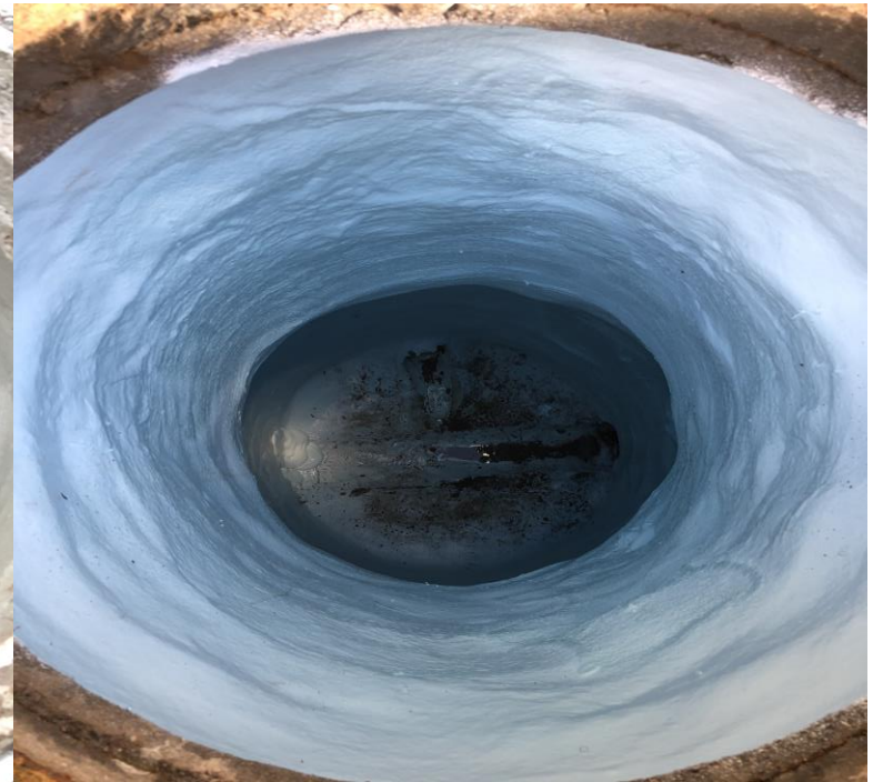
Wastewater Epoxies (250 Mil)
