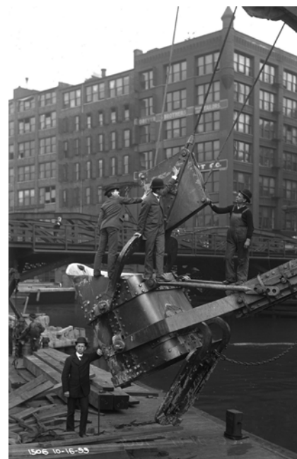
Workers pose on a dipper dredge bucket on October 16, 1899 during construction of a bypass channel on the South Branch of the Chicago River.
