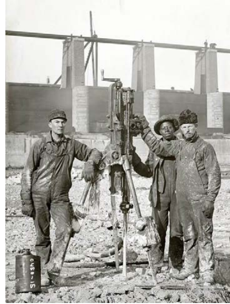
Three laborers posing next to a compressed air rock drill during the construction of the Chicago Sanitary and Ship canal. The estimated date is November 1896.
