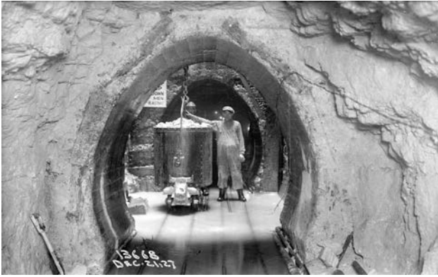
Workers with a hoist cage at the bottom of a drop shaft during sewer construction on December 21, 1927.
