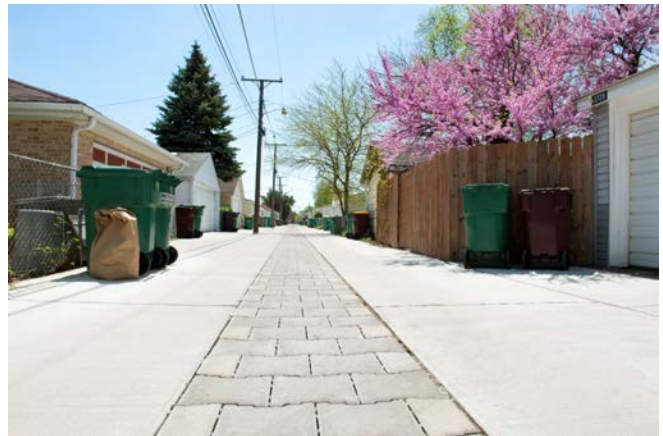
The District partners with local municipalities and other governmental organizations to fund Green Infrastructure projects that capture, store, and infiltrate stormwater by mimicking the natural water cycle. Funding is provided for construction projects that are in flood-prone areas and provide educational opportunities for residents on the benefits of Green Infrastructure. The 2019 Budget includes $10.7 million for cost sharing on local Green Infrastructure projects.
