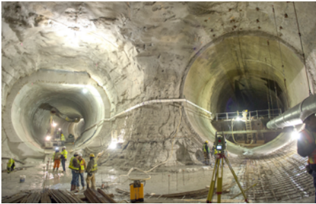
Construction at the confluence of the McCook Reservoir Connecting Tunnel (left) and Mainstream Tunnel (right)
