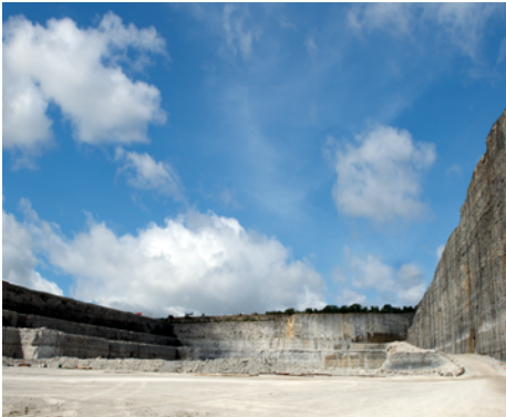
Thornton Reservoir, part of the Calumet TARP system, during excavation.
