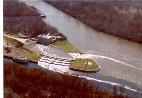
SEPA 5 at the Cal-Sag Channel and Chicago Sanitary and Ship Canal
