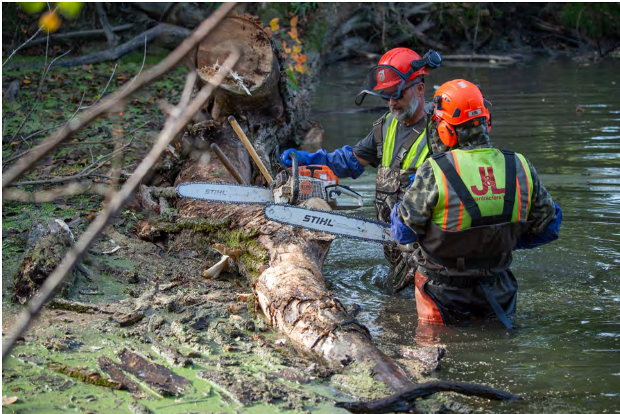
The MWRD's Small Streams Maintenance Program crew removes a large blockage in Watersmeet Woods in October on the Skokie River where the east and middle forks of the North Branch of the Chicago River meet near Winnetka.
