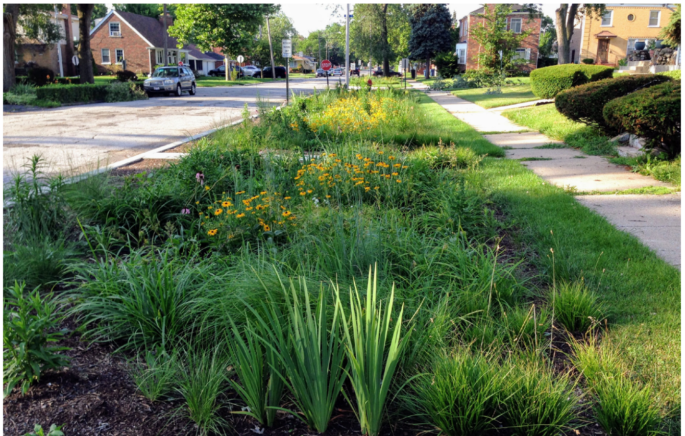
FIGURE 2.2 In a residential setting, a bioretention facility, seen here in Blue Island, can be an attractive landscape feature that also manages runoff from homes and streets.
