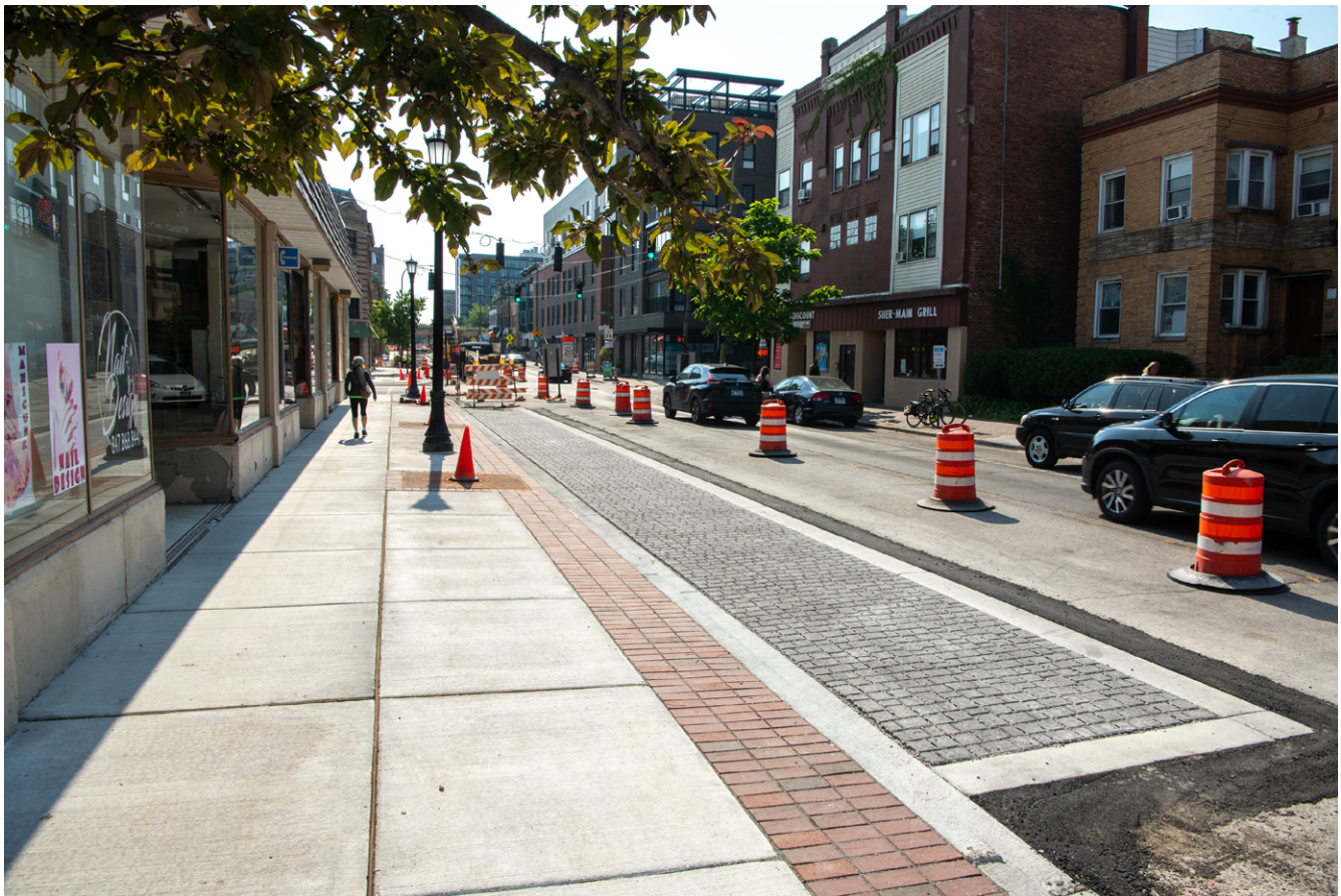
FIGURE 8.4 In a public right-of-way, permeable pavements are an effective solution for low-traffic residential streets.
