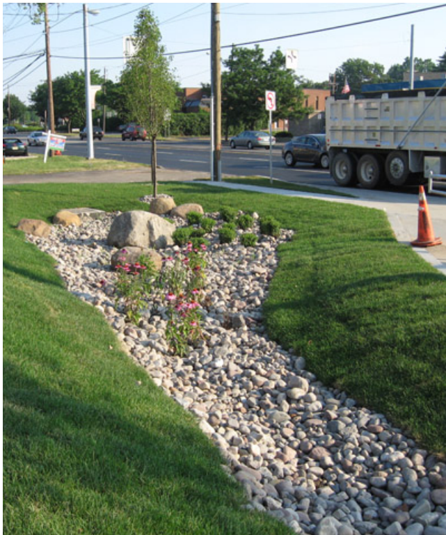
FIGURE 1.4 Filter strips (turf areas) surrounding an infiltration trench provide pretreatment in a public right-of-way.
