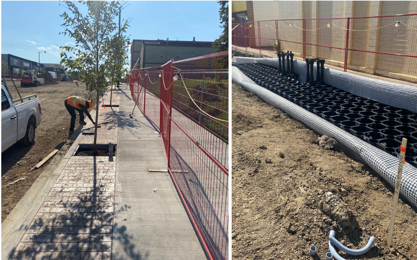
FIGURE 5.4 Stormwater trees optimize the public right-of-way by treating runoff underground. The trees utilize infrastructure like the modular soil cells shown here to reduce sewer strain while supporting a healthy urban canopy.
