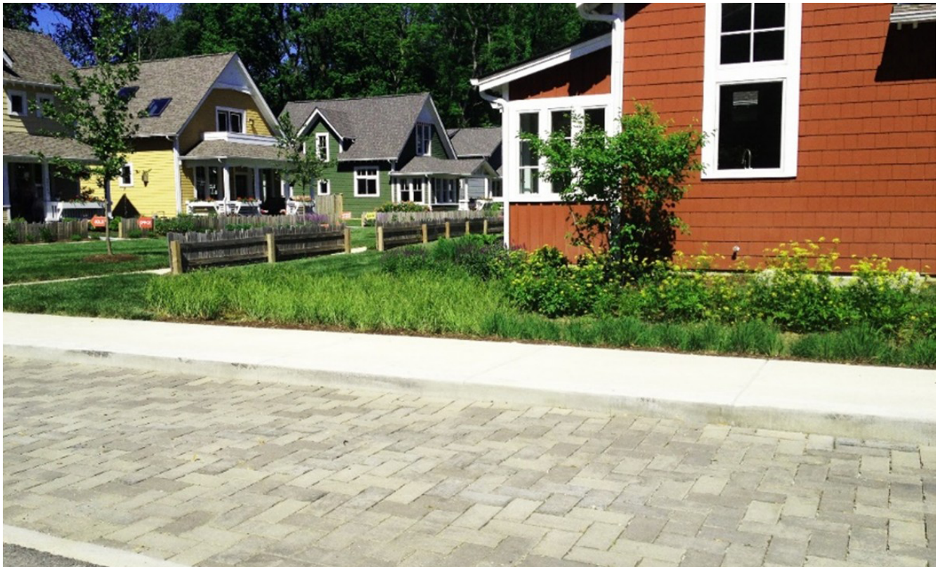
FIGURE 7.4 As part of a larger system, trenches can connect other green infrastructure practices to maximize site-wide infiltration. In this example, a network of infiltration trenches was installed beneath perimeter buffer bioswales, parking lane pavers, and common area bioretention areas.
