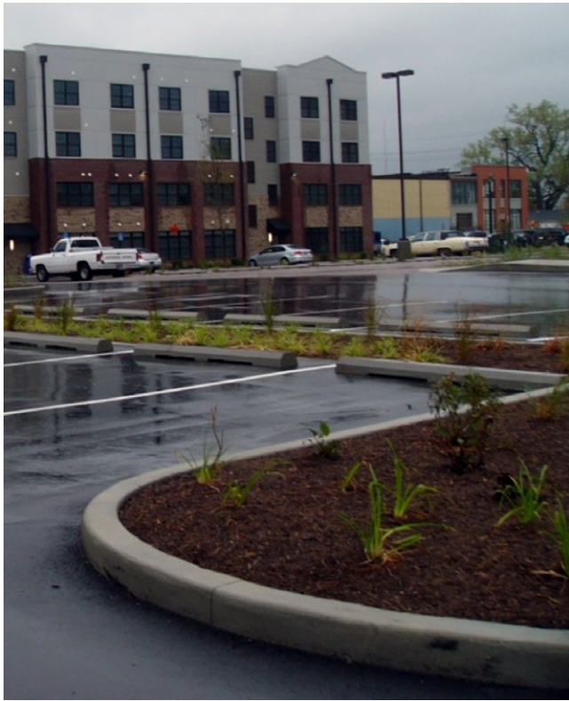
FIGURE 2.3 In commercial parking lots, bioretention islands can break up large expanses of pavement, treat runoff and help meet landscaping requirements.
