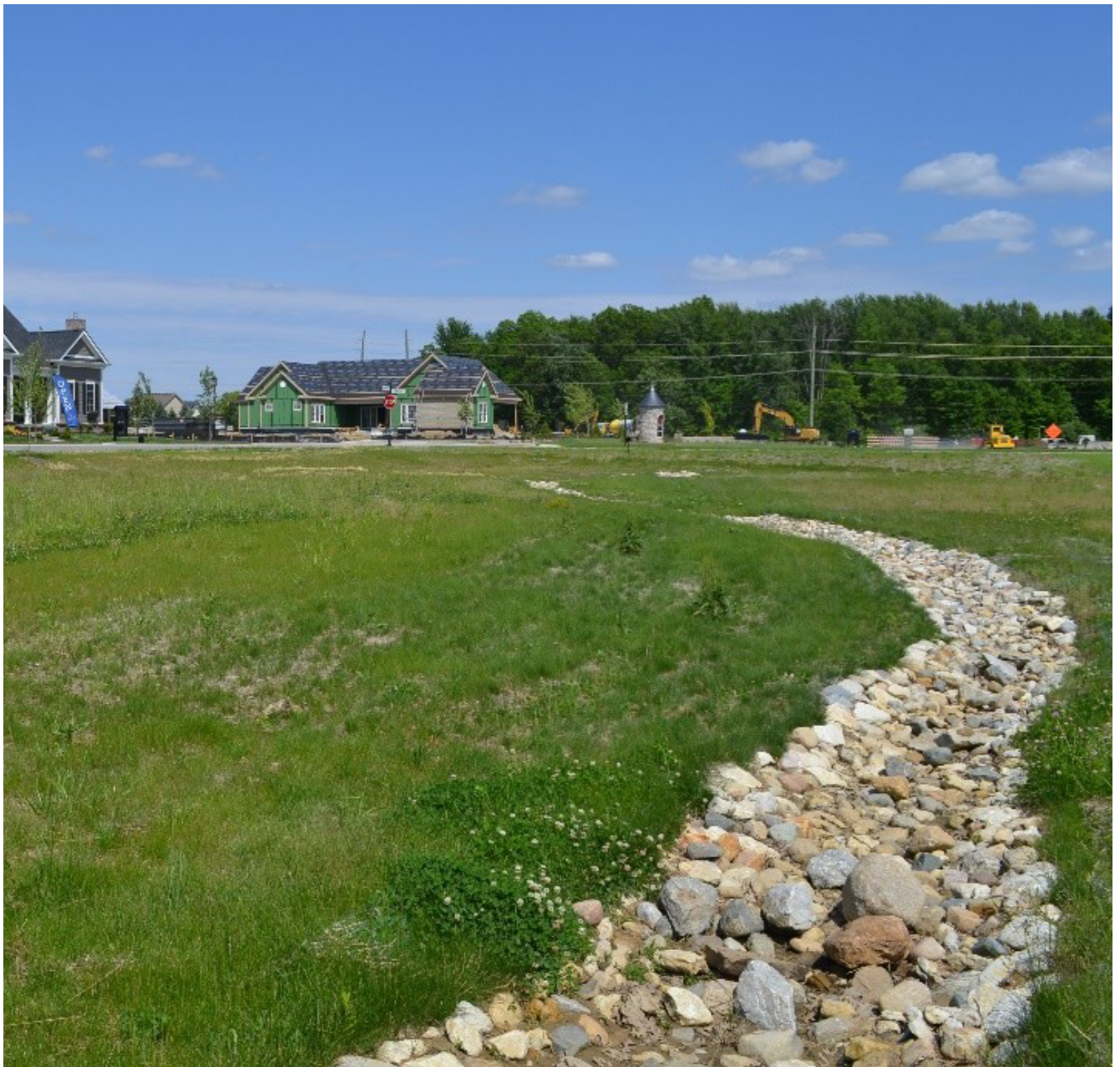
FIGURE 1.2 A vegetated filter strip (left of cobbles) provides simple, low-cost pretreatment for an infiltration trench in a new residential development.
