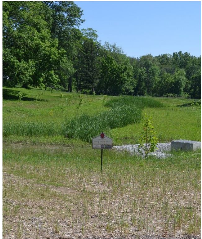
FIGURE 1.5 The surrounding filter strips provide pretreatment for a bioswale in an open space.
