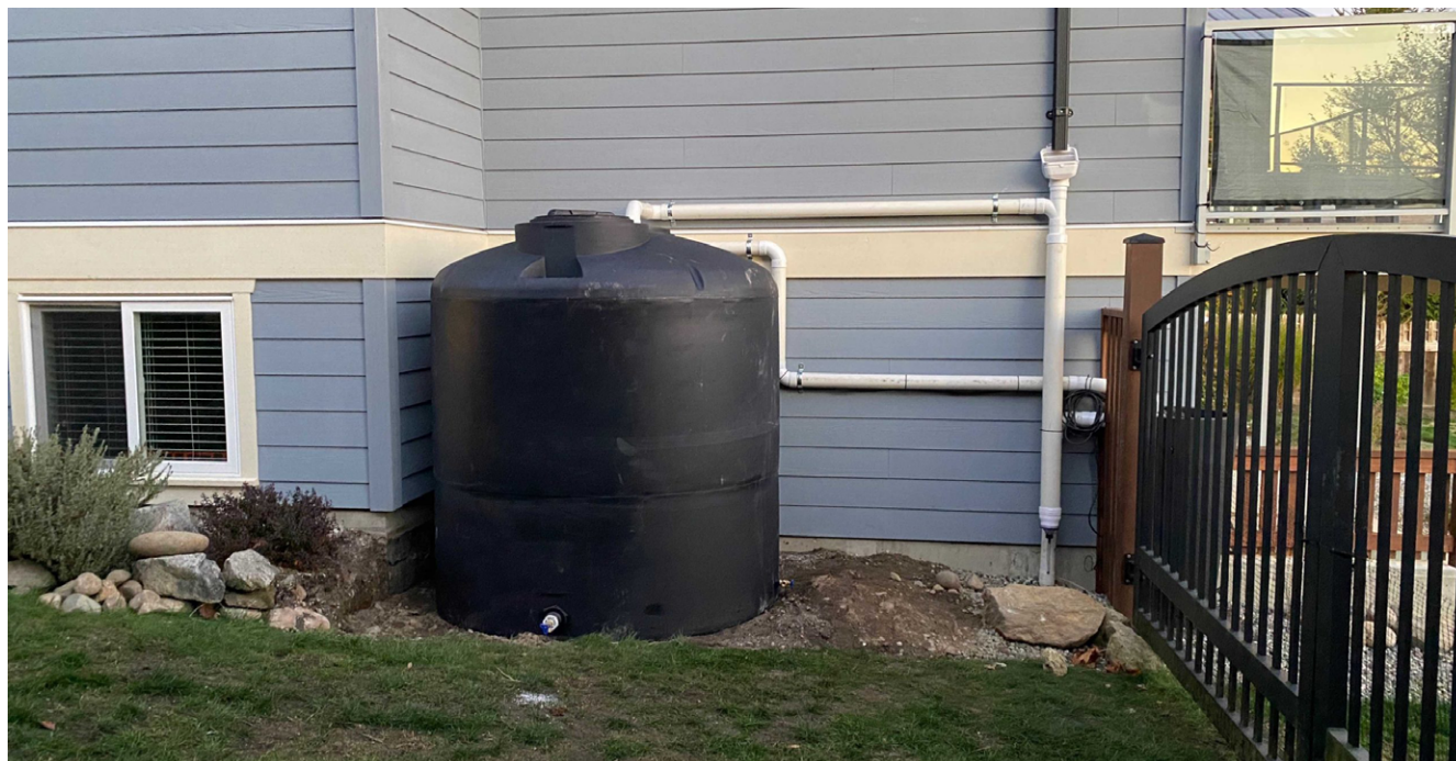
FIGURE 9.2 In a residential setting, a cistern can capture roof runoff for irrigating gardens and lawns.
