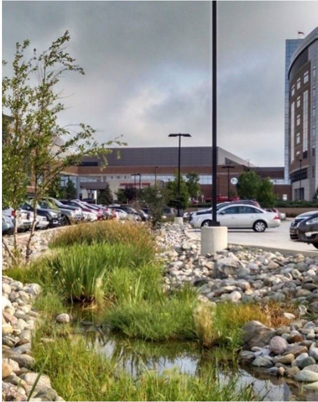
FIGURE 3.3 In a commercial parking lot, a bioswale serves as both a landscape island and a stormwater treatment feature.
