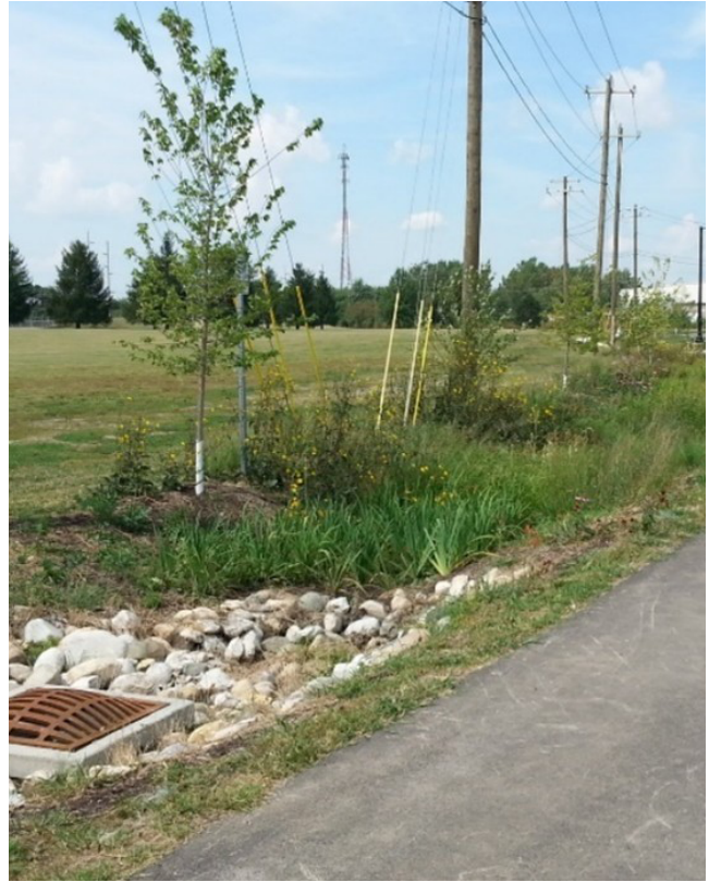
FIGURE 3.4 A simple bioswale in a public right-of-way (on the left side of the trail) provides drainage and treatment for road and trail runoff.
