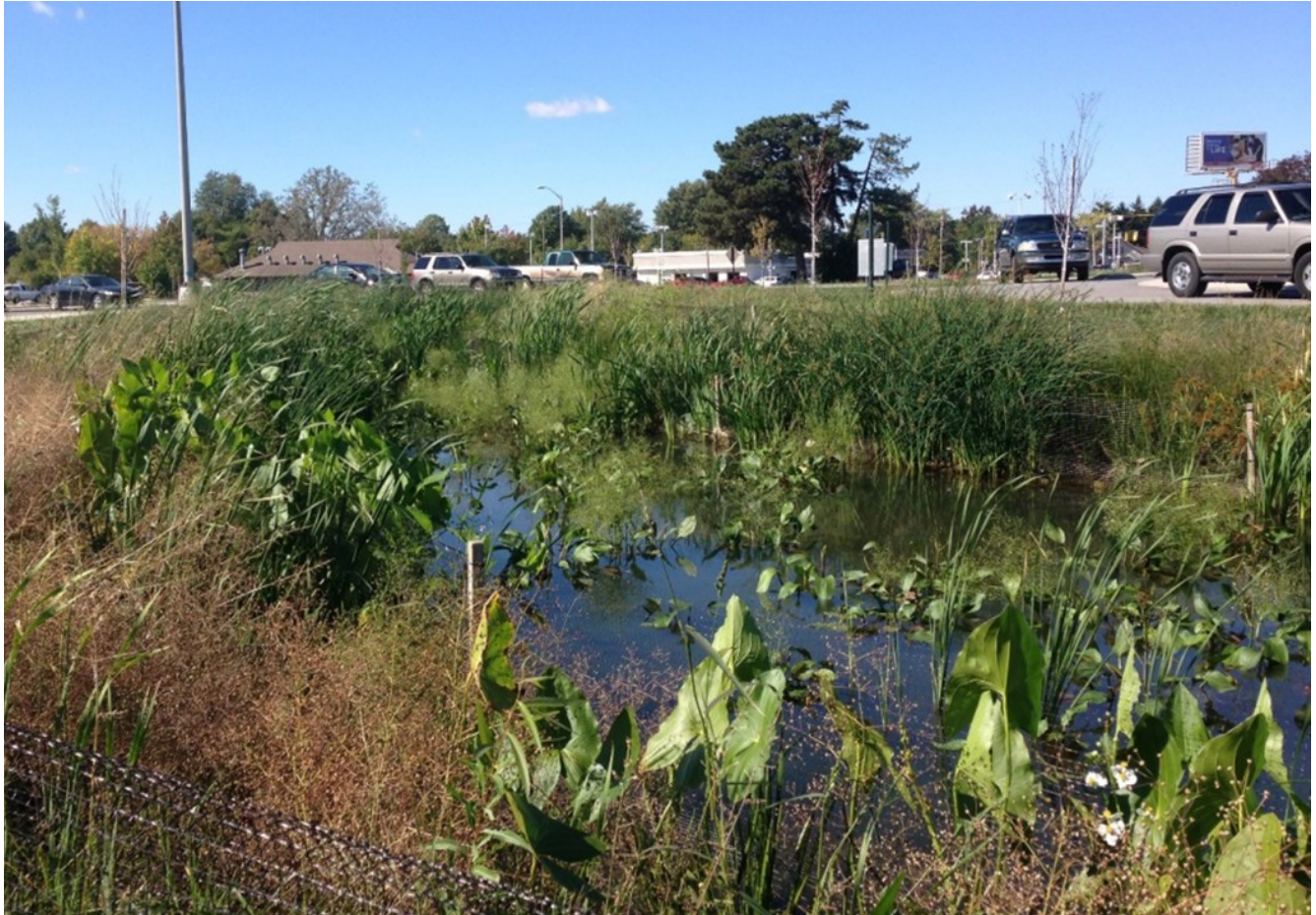
FIGURE 4.3 In a commercial area, a wetland can meet storage and landscaping requirements while treating parking lot runoff.
