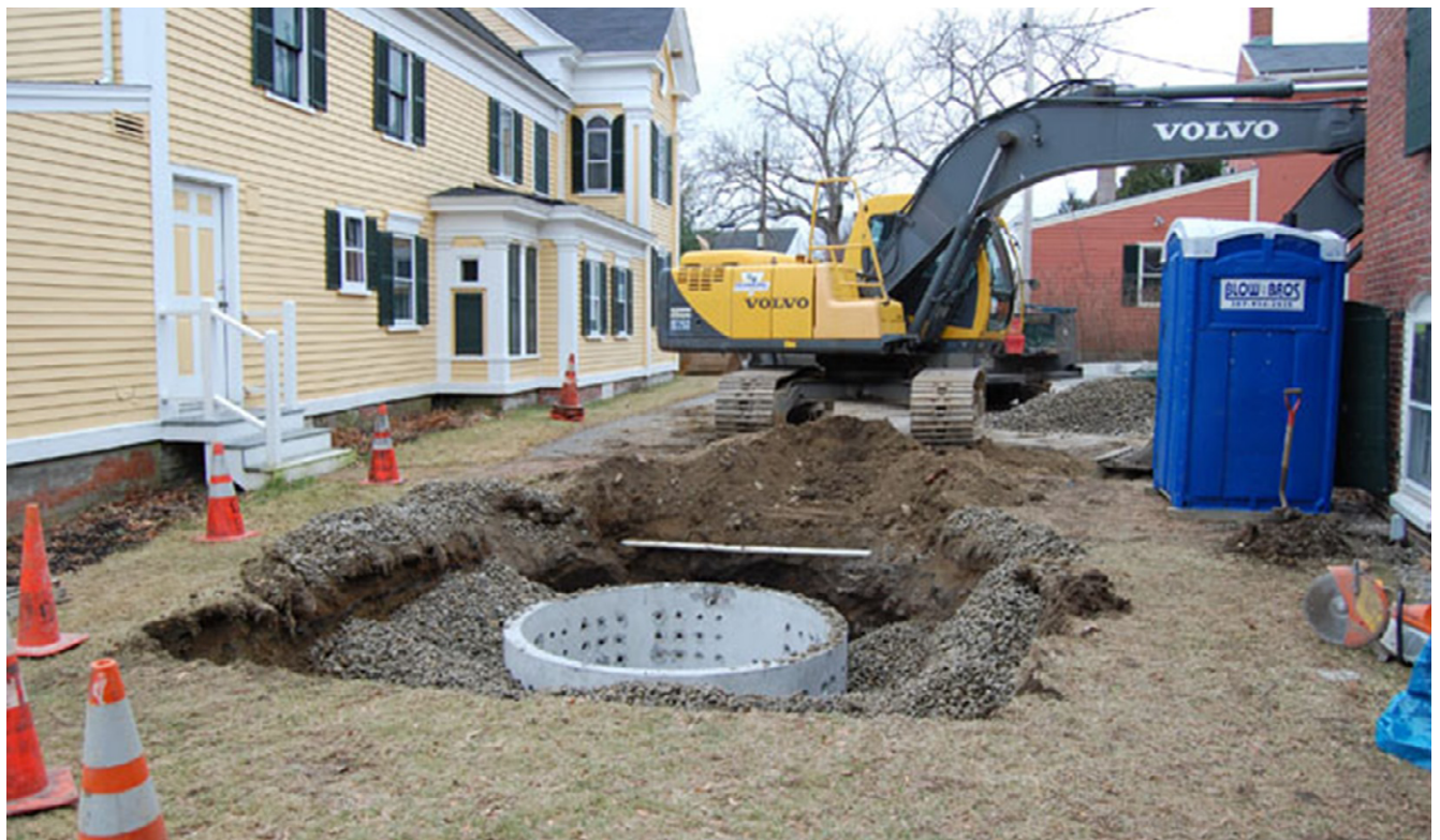
FIGURE 6.2 In a residential setting, a dry well can manage runoff from a roof or driveway, eliminating soggy spots in the yard.
