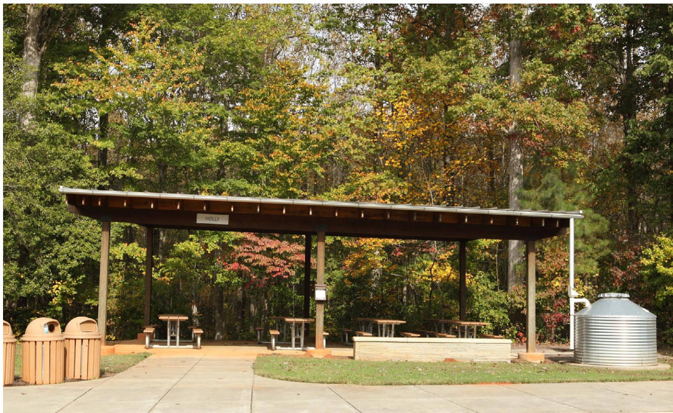
FIGURE 9.5 In a park, a cistern can capture runoff from a shelter roof to irrigate nearby landscape beds or athletic fields.
