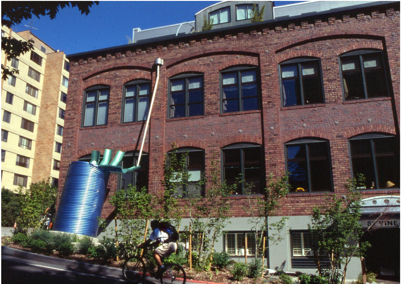
FIGURE 9.3 In a commercial area, a large cistern can supply water for irrigation.
