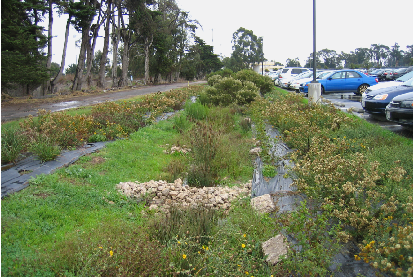
FIGURE 1.3 A filter strip provides pretreatment for a bioswale in a commercial parking lot.
