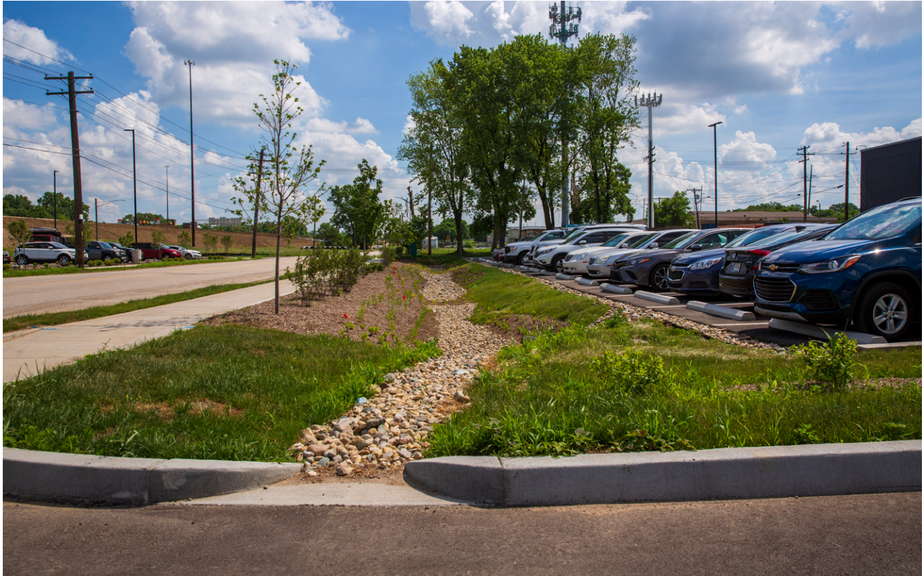
FIGURE 7.3 Located at a light industrial site, this infiltration trench captures and treats runoff from the adjacent parking lot and public right-of-way.
