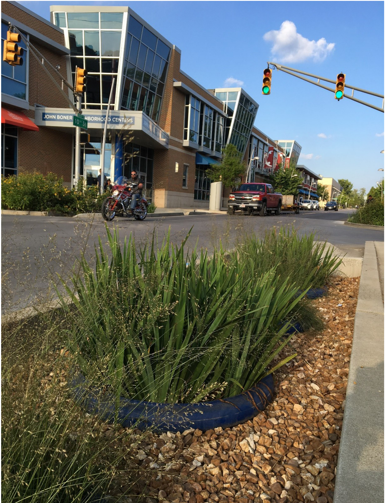
FIGURE 6.3 In a public right-of-way, dry wells can be installed to capture street and sidewalk runoff without disrupting pedestrian flow. In the photo, dry wells are integrated within a bioretention area to create a hybrid system.
