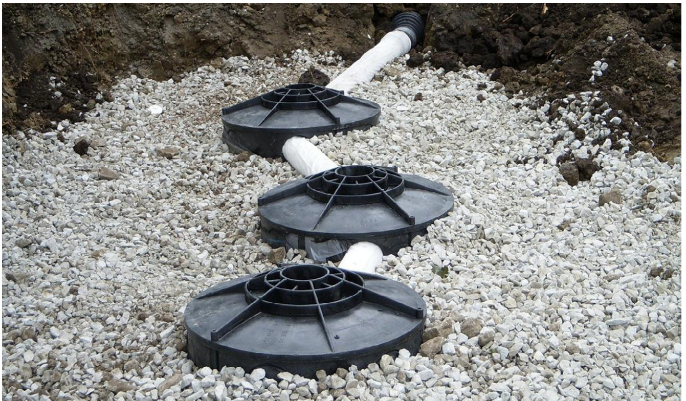
FIGURE 6.5 In parks or open spaces, a series of smaller dry wells can be used to address localized drainage issues without disturbing large areas.
