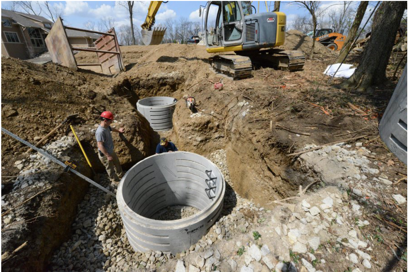
FIGURE 6.4 In a commercial site, a series of large dry wells can be installed under parking lots or landscaped areas to meet storage requirements.
