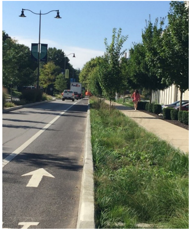
FIGURE 2.4 Along roadways, bioretention facilities can treat runoff, calm traffic and increase the capacity of existing sewer systems.
