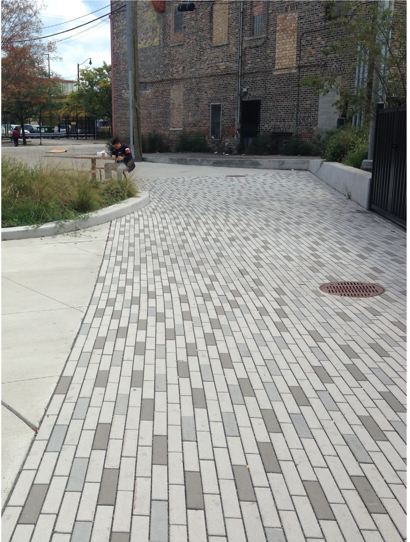
FIGURE 8.5 Permeable walkways and patios are ideal for parks and plazas, reducing runoff while providing durable, attractive surfaces.
