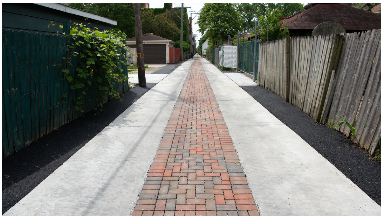
FIGURE 8.2 In a residential setting, permeable pavers in a parking lane, driveway or alley can manage runoff while enhancing the aesthetics of the neighborhood.
