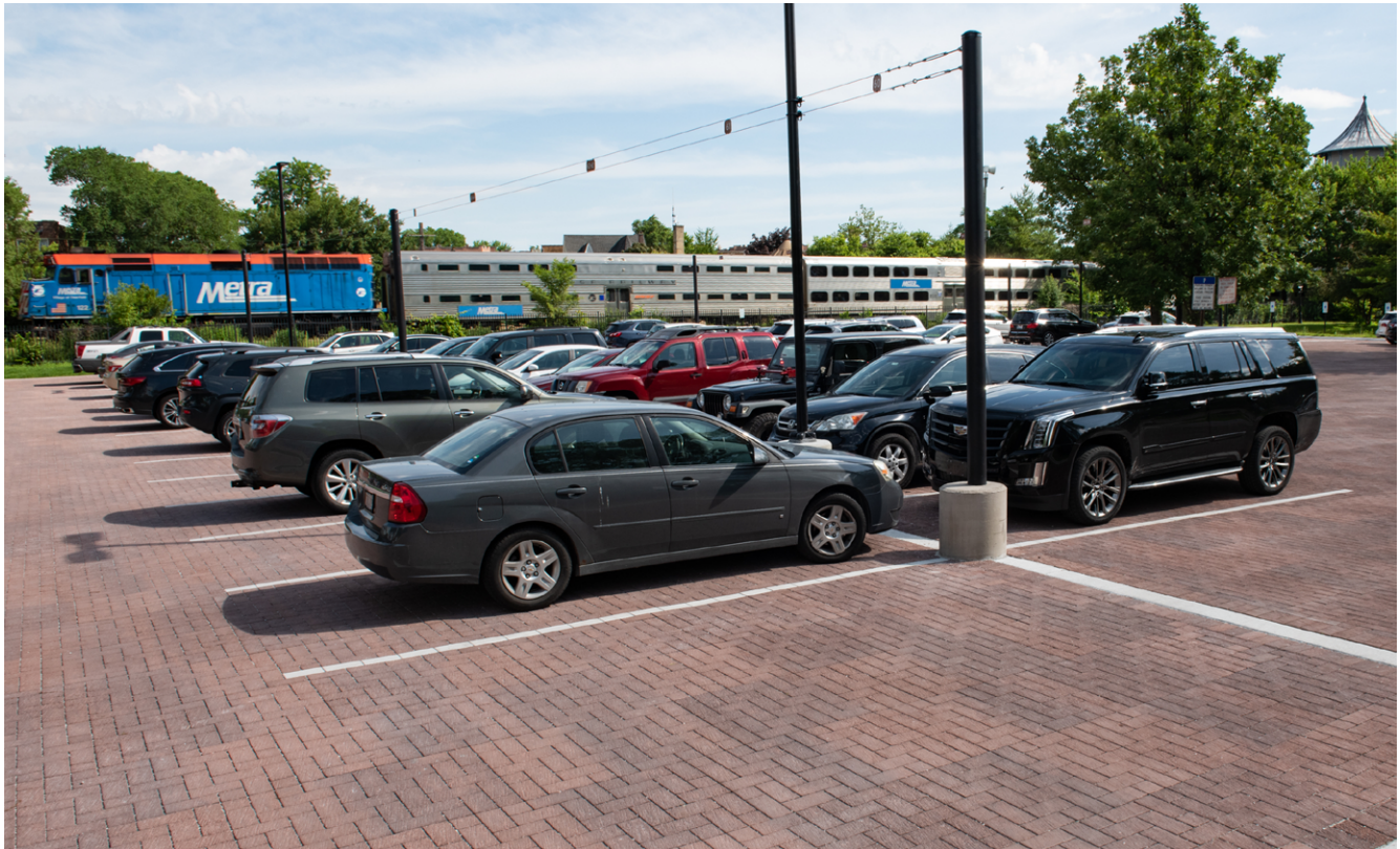
FIGURE 8.3 In a commercial area, a fully permeable parking lot maximizes stormwater storage and reduces runoff, capturing water on location and protecting area water quality.
