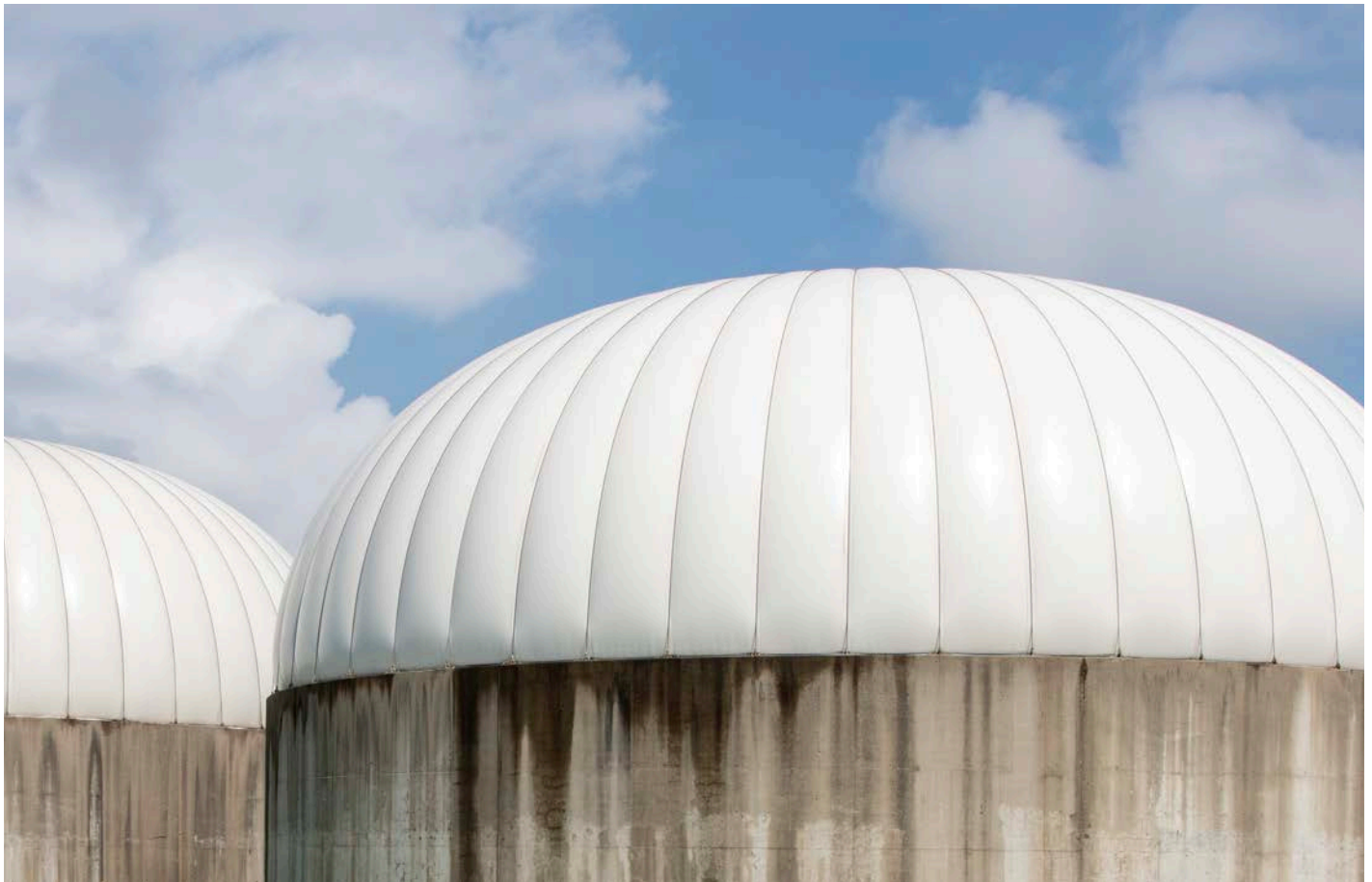
ABOVE Anaerobic digesters at Egan Water Reclamation Plant produce biogas that the MWRD harnesses to produce electricity, recover heat, and reduce energy demands.
