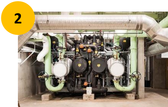
Collection system sewer thermal recovery
