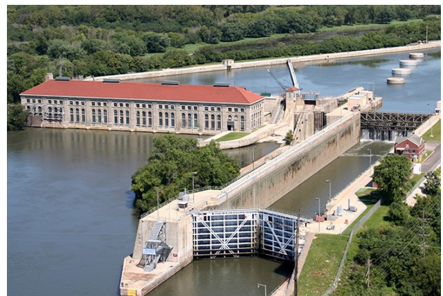
Lockport Powerhouse and Controlling Works. The Lockport Powerhouse generates approximately 40 million kilowatt hours of electrical energy annually, generating $1.2 million in revenue for the District.
