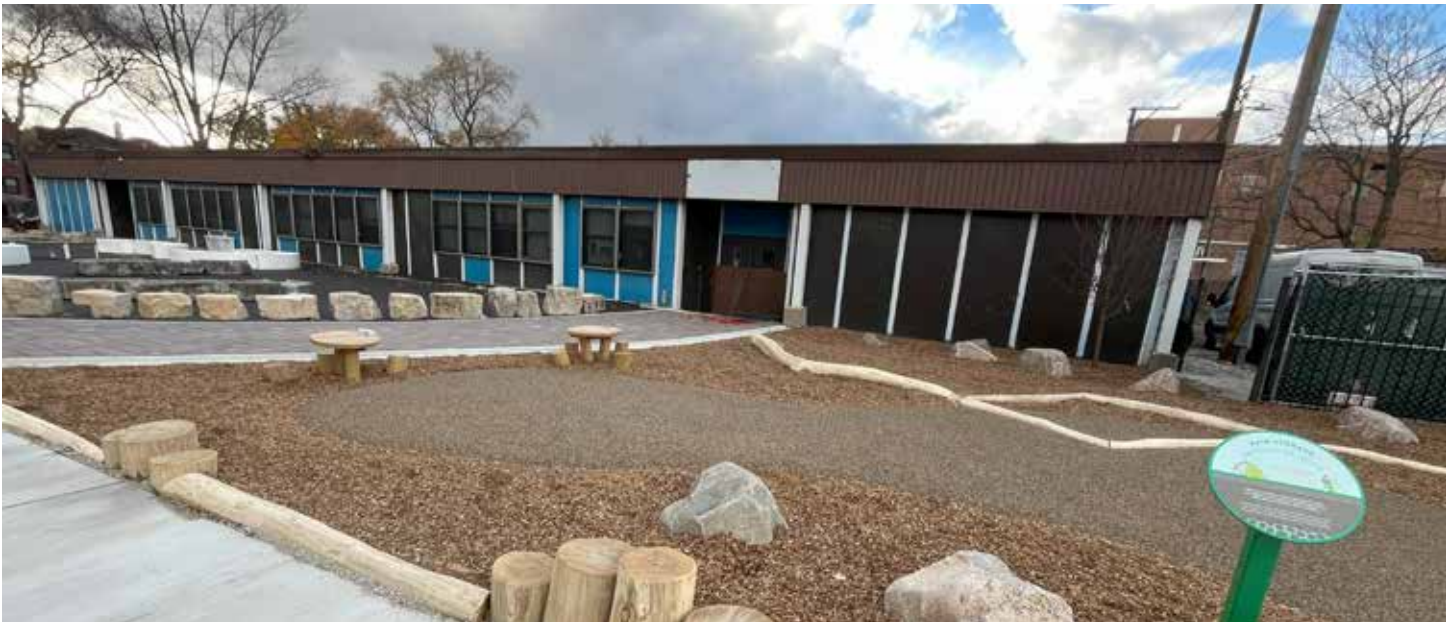
With its new turf field, permeable paver plaza, permeable play surface and rain gardens, the schoolyard at Spencer Elementary Technology Academy in Chicago's Austin neighborhood can capture approximately 190,000 gallons of stormwater, thanks to the MWRD's Space to Grow partnership.
