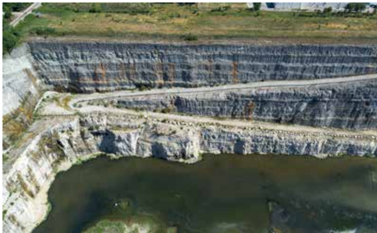
An entrance ramp along the north side of the MWRD's Thornton Composite Reservoir during near empty conditions demonstrates the scale and detail of excavation operations to carve out a reservoir from limestone and provide enough capacity to contain up to 7.9 billion gallons of storage.
