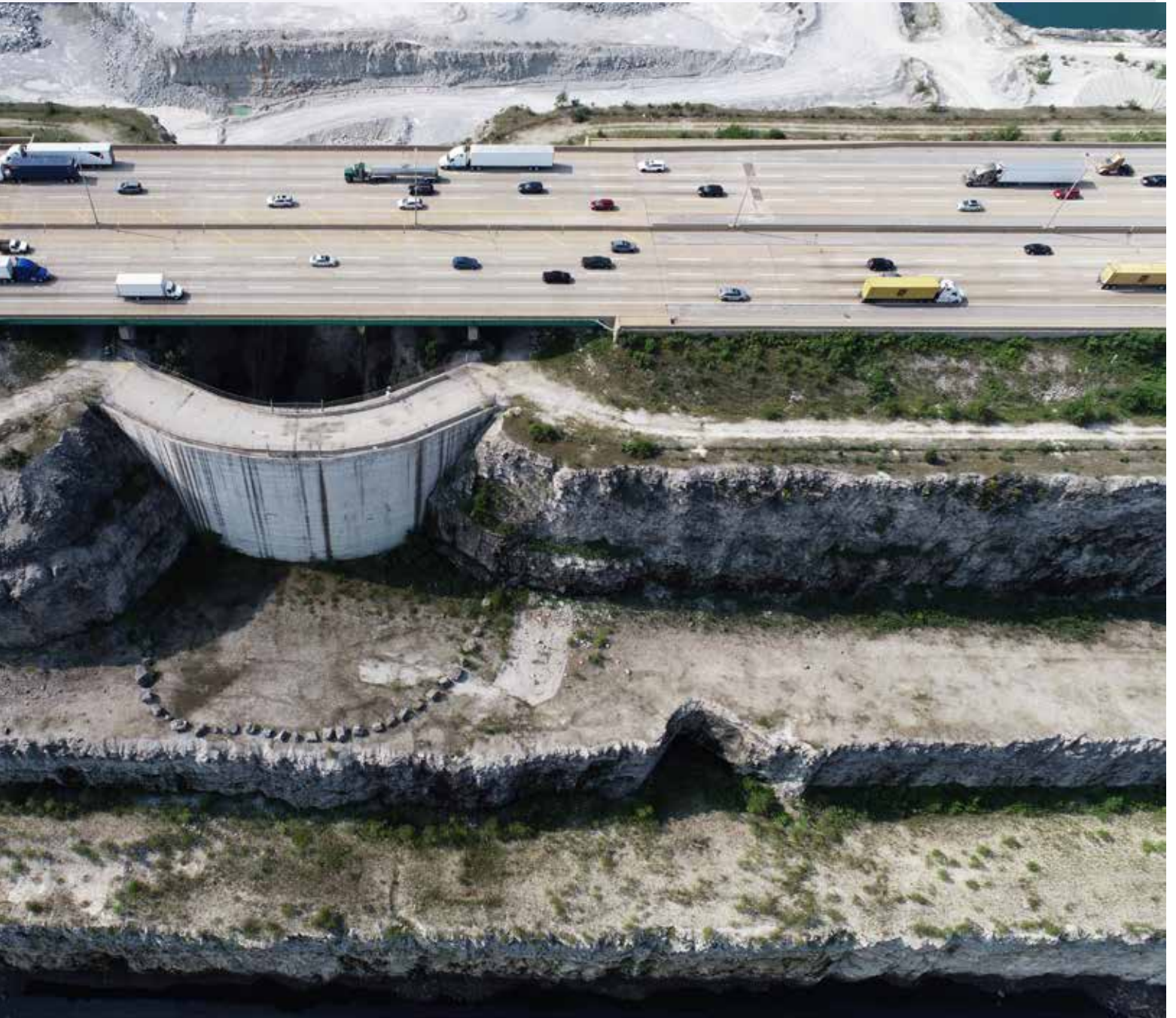
Vehicles on the Tri-State Tollway (I-294) pass over a concrete dam made of roller compacted concrete that seals an old mining access road and sits high atop the MWRD's Thornton Composite Reservoir designed to provide up to 7.9 billion gallons of storage.
