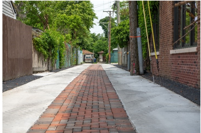
According to the District's Green Infrastructure Partnership Program, permeable alleys are more attractive and hold more stormwater. The District and municipal partners completed several green alley projects, as shown above in Maywood.
