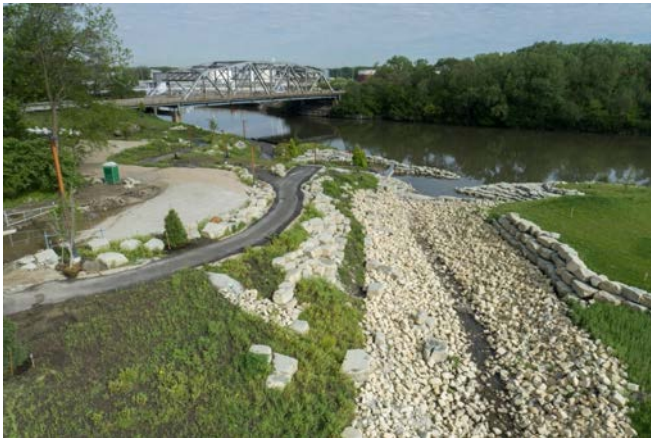
The diversion channel for the Midlothian Creek Flood Control Project in Robbins that the District helped fund is an example of a stormwater partnership project directly supporting municipalities in Cook County to address localized flooding and drainage concerns.
