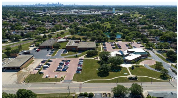
Six new green parking lots using permeable pavers to collect more stormwater and reduce the load on local sewers and waterways can be seen at North Riverside Commons complex.
