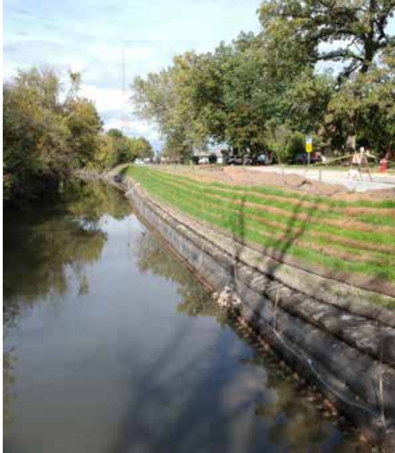
▲ Streambank Stabilization along Addison Creek - North Riverside/ Northlake, 14-108-3F
