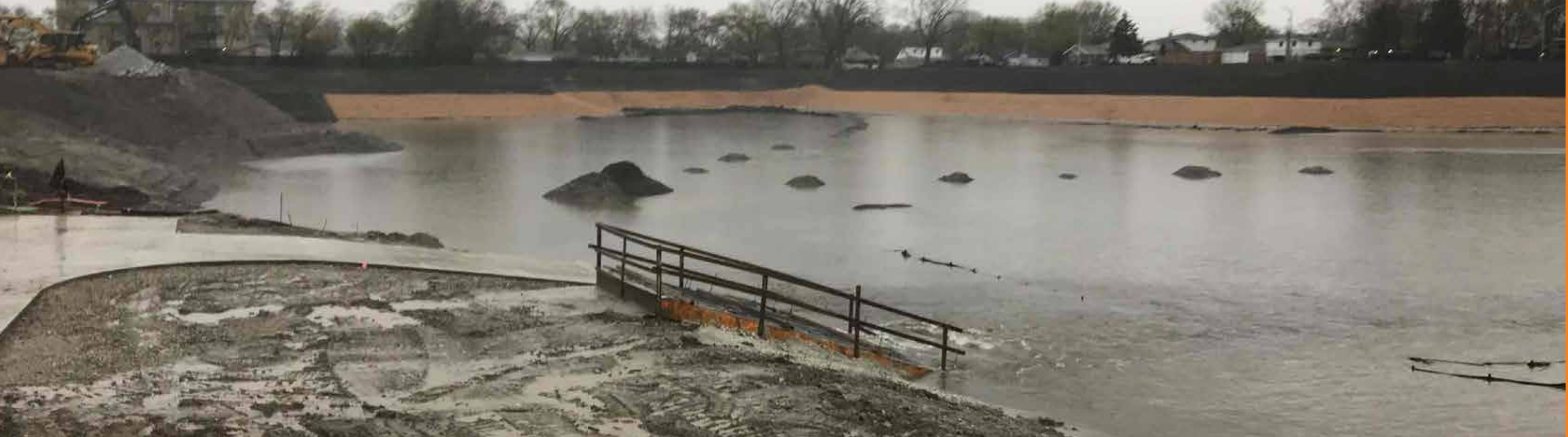
▲ Melvina Ditch Reservoir Improvements, 14-263-3F
